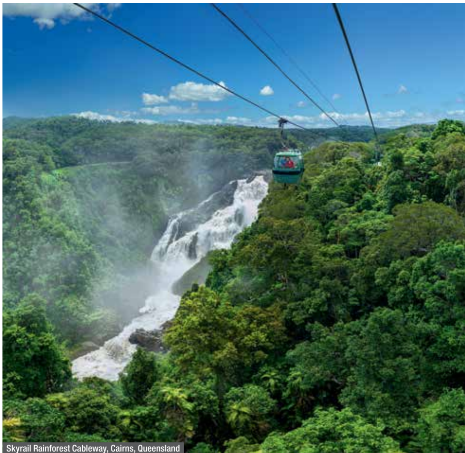
Skyrail Rainforest Cableway, Cairns, Queensland
